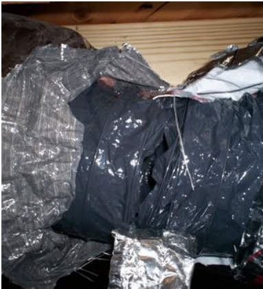
Improperly installed heating and cooling systems can reduce system efficiency by 30 percent and can be dangerous
